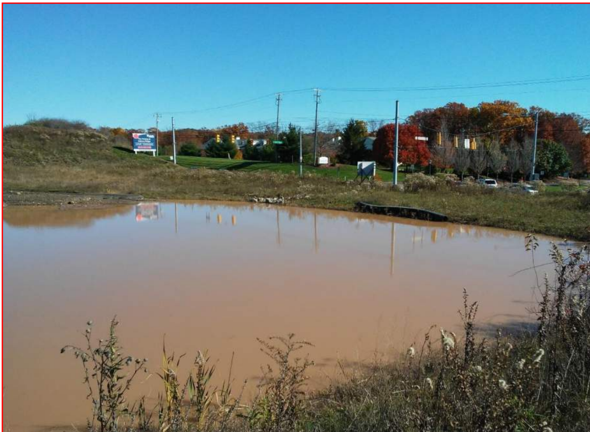
Photo 15: Stormwater sediment basin with leaking embankment facing east (11.8.17)
