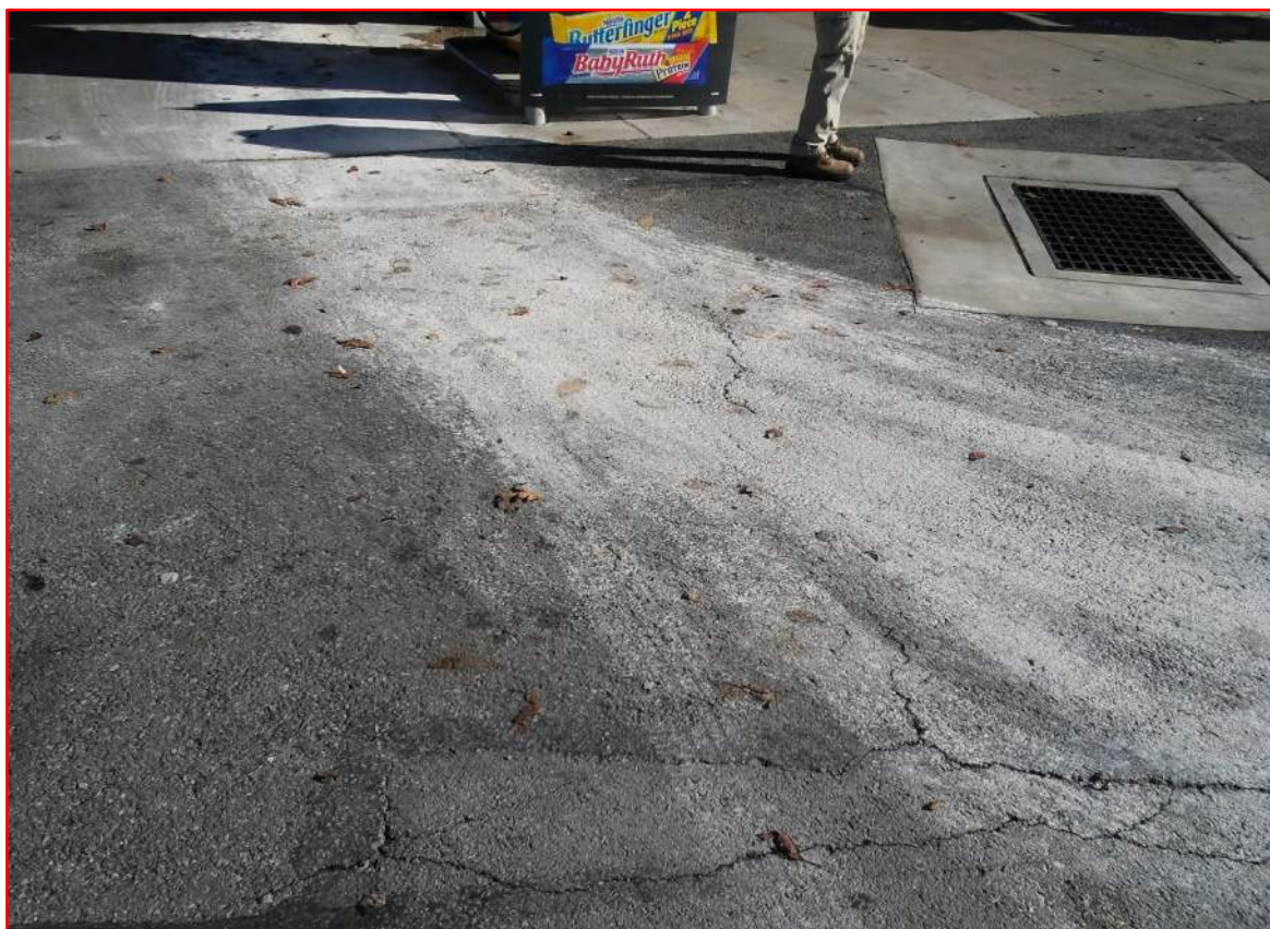
Photo 14: White absorbent material and inlet with sheen in Sunoco parking lot (11.8.17)
